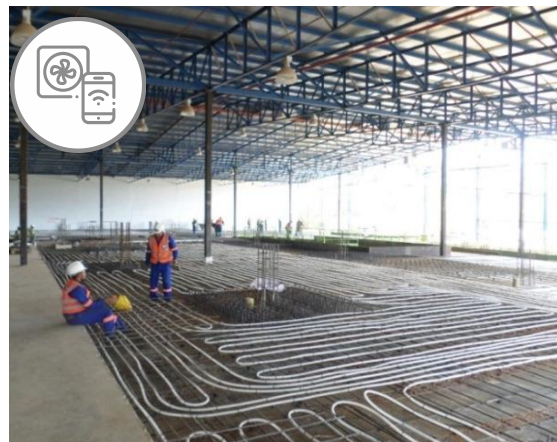
In slab heating and cooling
